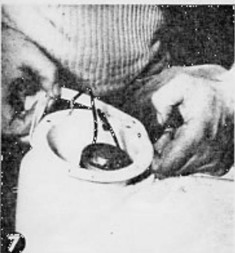
7 Install gasket, locate to proper hole position. Install four cartridge mounting screws, tighten so that gasket seals between motor housing flange and tank body opening.
