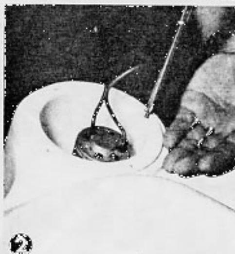
2 Remove four cartridge mounting screws.
