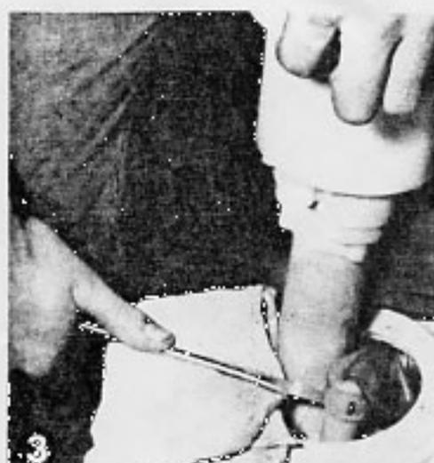
3 Pull cartridge assembly upward until hose connection is exposed. Protect plastic tank body with folded cloth and pry off hose connection with screwdriver.
