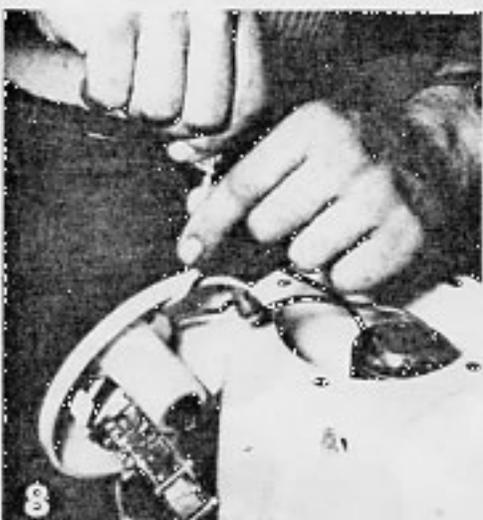
8 Reconnect electrical wires, twisting in a clockwise direction. Screw on plastic connection insulators.
