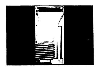
The sealed combustion unit contains a mixture of ammonia, water and **a** rust inhibiting agent. After this solution is introduced into the coils, this unit is pressurized with hydrogen gas. When this system is in operation, the ammonia vaporizes in the hydrogen atmosphere and absorbs heat from inside the refrigerator.
